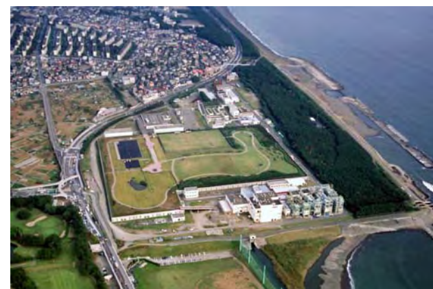
Yanagishima sewage treatment plant
