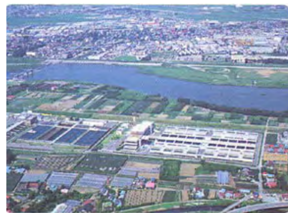
Samukawa water purification plant
